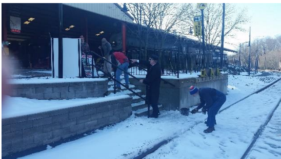
Clearing the Roberts platform and stairs.
